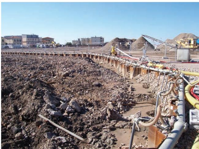
Fig. 6 - Groundwater dewatering system.
